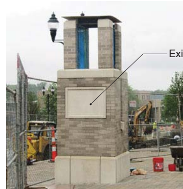
Reference Photo (Pillar Under Construction)
